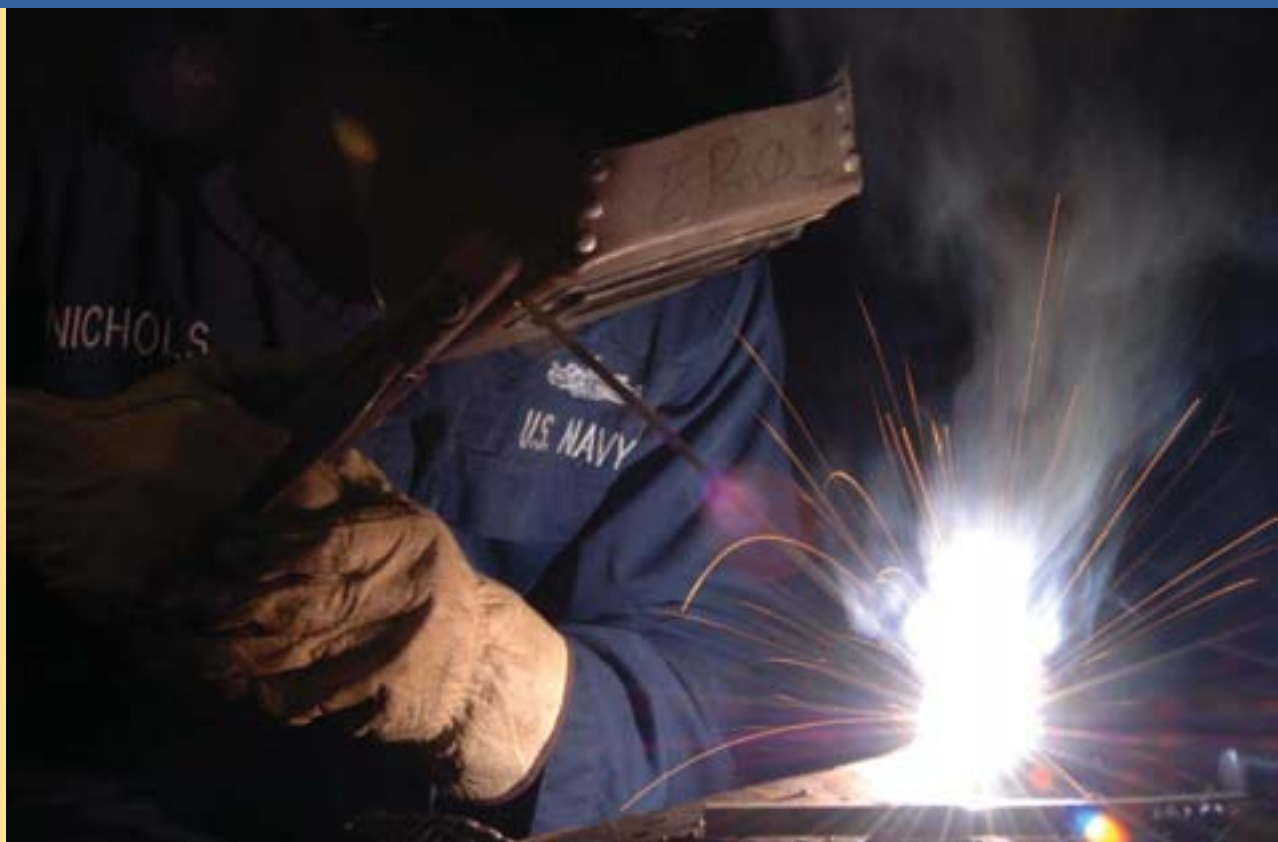
Hull technician welds ship stanchion (Image Courtesy of U.S. Navy)
