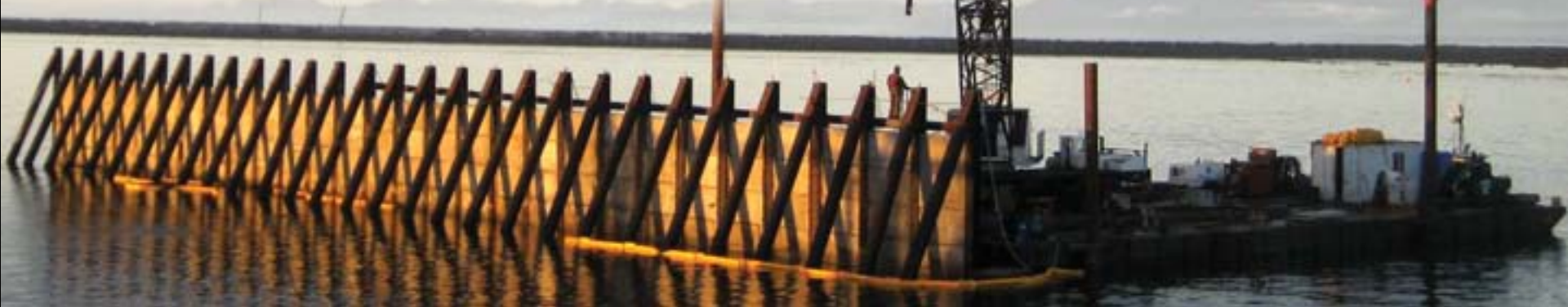
Neah Bay Bulkhead during construction
