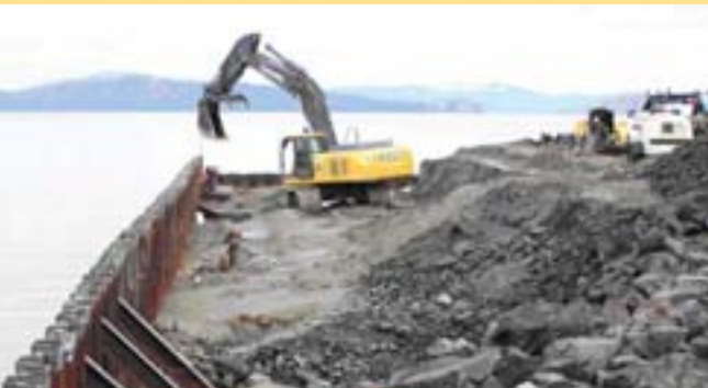
Tongue Point Bulkhead, west seawall (Image Courtesy of U.S. Coast Guard)
